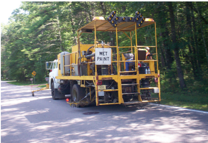
A Shawano County Highway Department truck paints white stripes along the side of Cloverleaf Lake Road. A donation from the Stockbridge-Munsee Tribe paid for the safety measure on several town roads.
